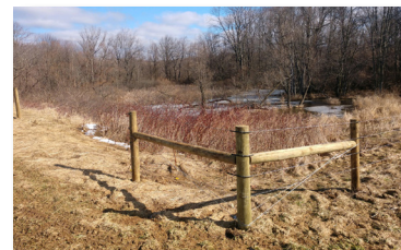
Wetland Exclusion Fencing
